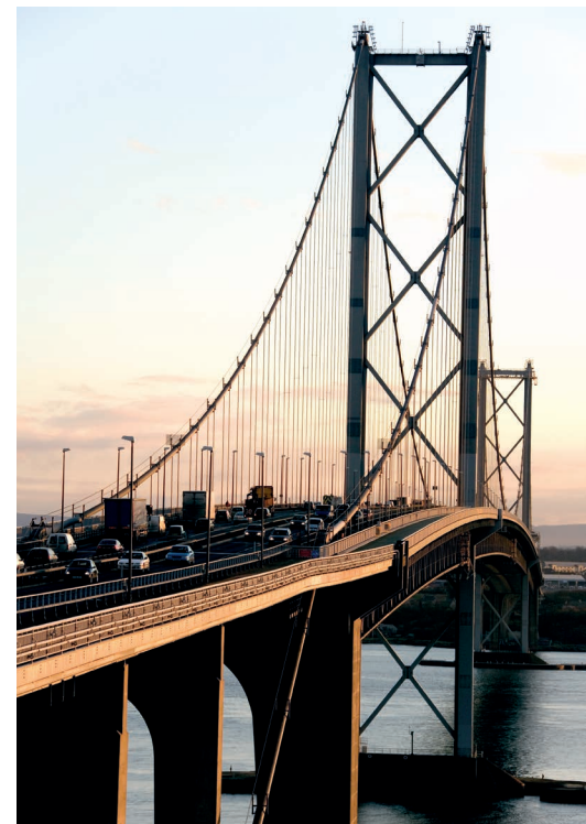
8power's device was tested on the Forth Road Bridge.
