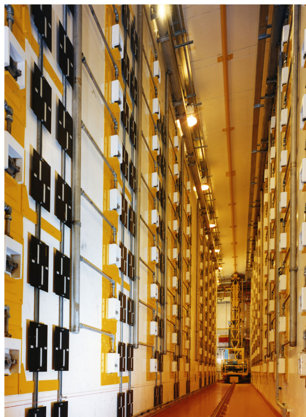
Fig. 1 Sellafeld plutonium product store. View of the interior of a Sellafeld plutonium product store (reproduced with permission of the copyright holder, the Nuclear Decommissioning Authority).
