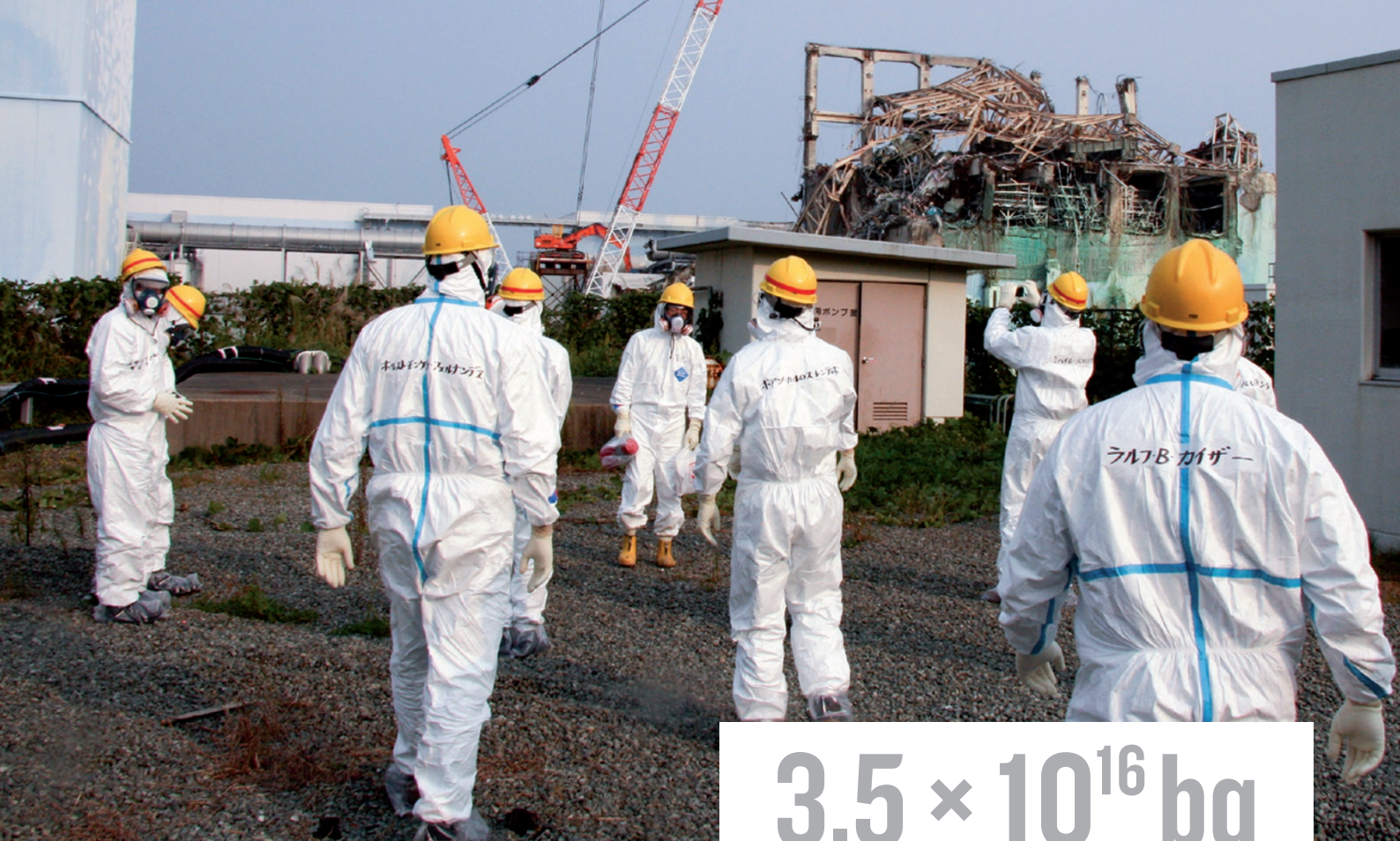
Fallout: inspectors take stock of the damage to Fukushima Daiichi.
